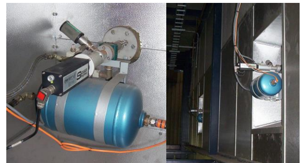
Pyrometer with air purge tube and shock blower
