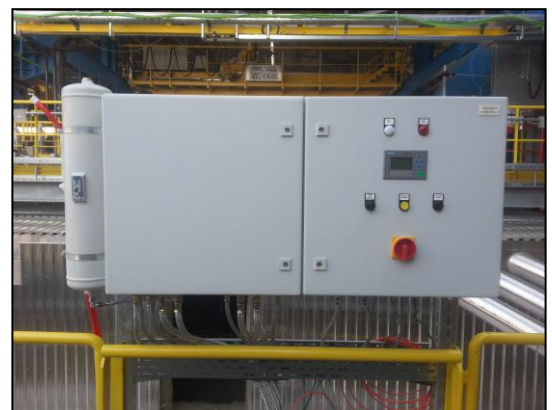
Infrared-Camera "PYROINC Flamefilter" with automatic transfer device and cabinets on boiler top
